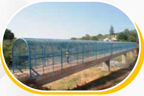
Completed Marite pedestrian bridge signifies the Provincial Infrastructure Plan coordinated by OTP.
