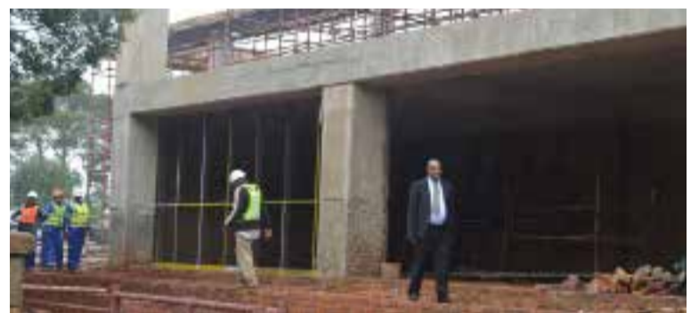
Dipaleseng Executive Mayor, Cllr Mafunda Makhubu inspecting the building under renovation.
