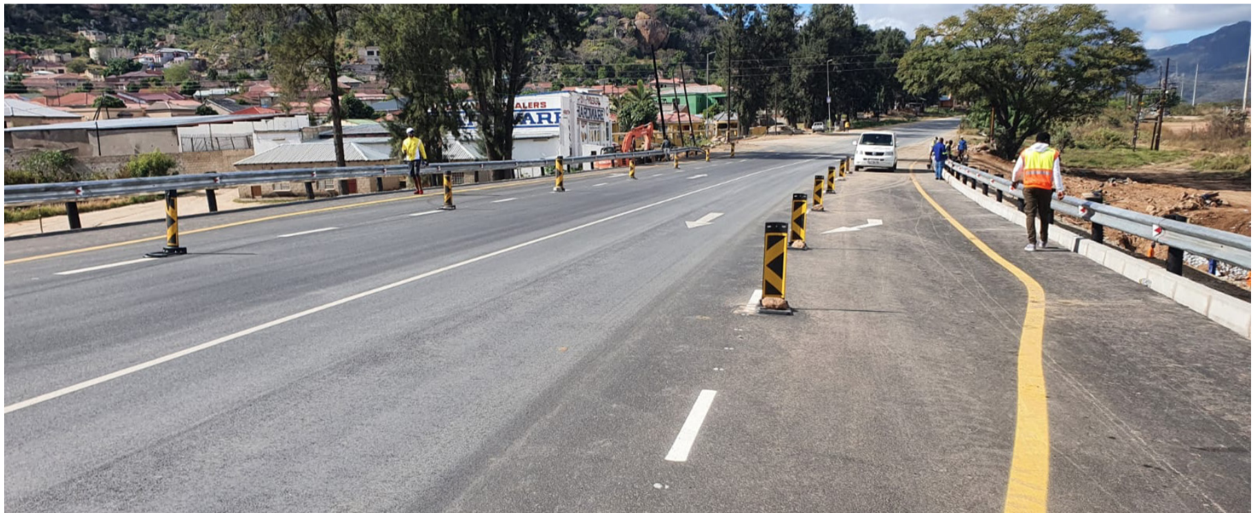
New look Tekwane South bridge that connects Kanyamazane and Mbombela.
